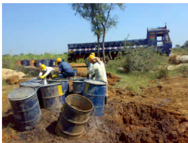
Fig. 2. Removing of waste from Koratagere dump site
