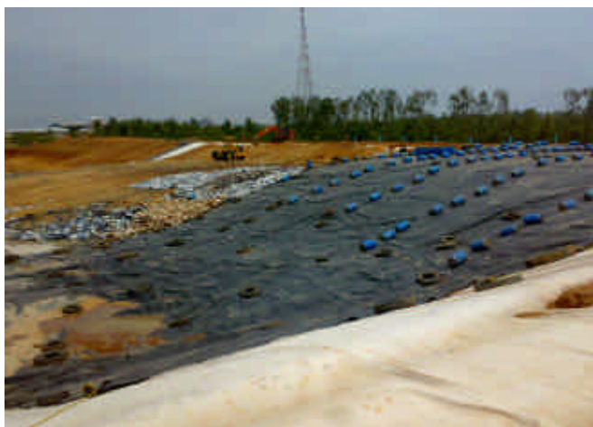
Fig.1 Land fill facility at Dabbaspet
