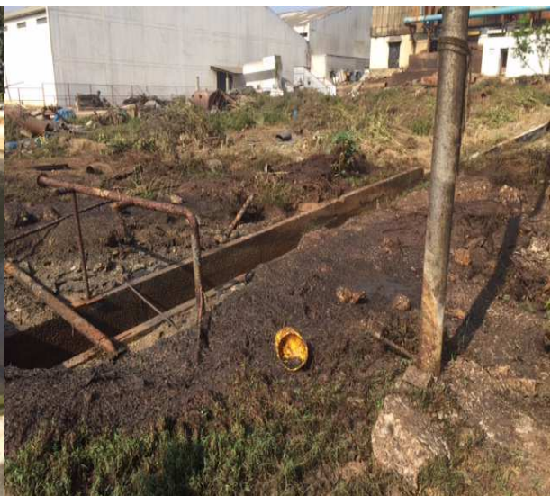
Effluents carrying drains
