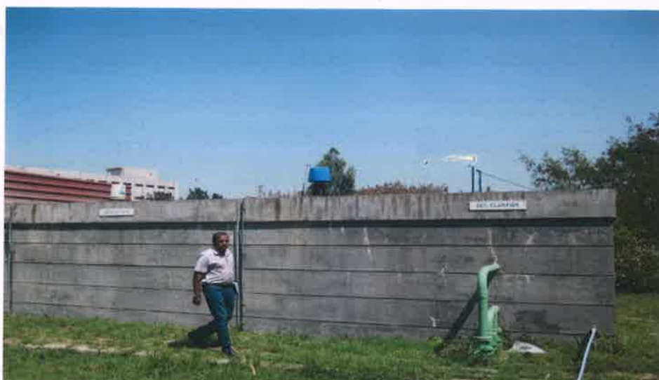
View of STP
