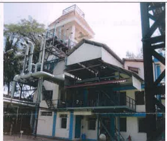
View of Plant Area
